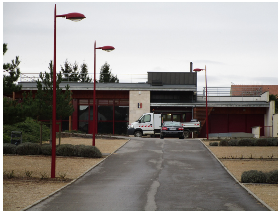
Figure 24 : le foyer rural
